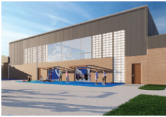
Cuyahoga Valley Christian Academy Weight Room Renovations
