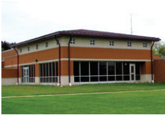
Jackson Local Schools Lake Cable Elementary Addition + Renovation
